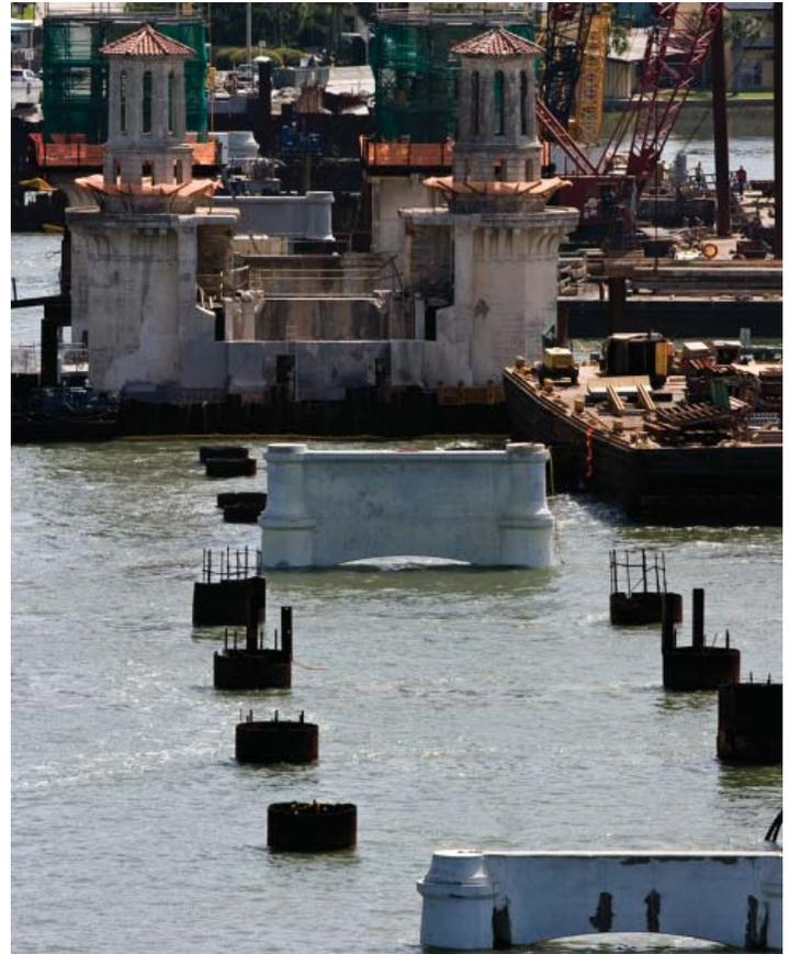
A series of drilled shafts reinforced with steel casings at the Bridge of Lions rehabilitation project, St. Augustine, Fla., 2008
