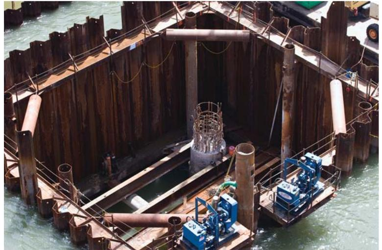
Close-up view of a drilled shaft pier surrounded by a cofferdam that protects the area from water intrusion during construction, Bridge of Lions rehabilitation project, St. Augustine, Fla., 2008
