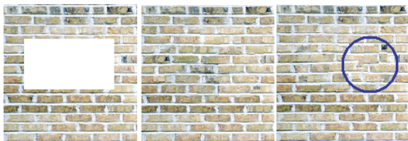
Figure 3: Left: Images of a wall with a missing part. Middle: The result using the graphcut updating method. Right: The result using the direct updating method. There is noticeable structure discontinuity inside of the blue circle area.
